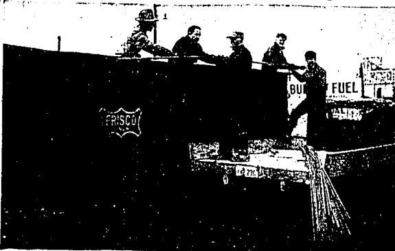
Burley Jaycees and city employes unload reinforcing steel obtained for use in constructing the new Burley swimming pool. Don Gray, second from left, is chairman in charge of assembling materials for the pool. The steel was the first material obtained. (Photo by Cassida Steelmith-Staff engraving)
