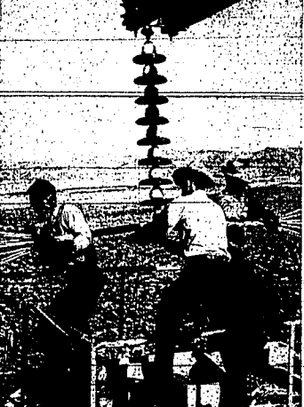
Working on a 33-foot mobile tower, an Idaho Power company quickly twists armor rods onto the inch-thick electric line to protect it from friction and vibration. The man in the center is attaching the line to the string of insulators suspended from the pole structure. Men with headphones direct the driver of the truck to lower or raise the tower, move forward or backward so the platform is just right for efficiency of workmen. (Idaho Tower photo—staff engraving)
