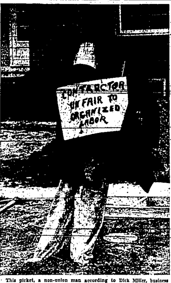
This picket, a non-union man according to Dick Miller, business agent of the striking local carpenter's union, was discovered standing in front of a construction project on Second avenue.
