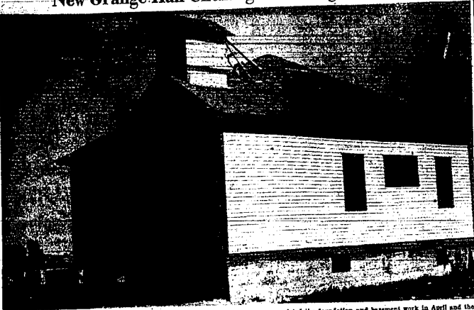
The old Park Lane schoolhouse which has become the new home of the Twin Falls Grange is shown above on the recently built foundation south of Twin Falls on Lux Lakes boulevard south. Members of the
