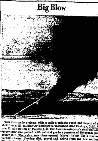
This man-made cyclone with a mile-a-minute speed and impact of a shell from a 105-millimeter howitzer is unleashed near Coalinga, Calif. A new 12-in. section of Pacific Gas and Electric company's steel pipeline "super inch" was packed with natural gas to a pressure of 500 pounds per square inch. The valve, was then opened (above) to act like a reverse vacuum cleaner, blowing dirt, gravel and debris from the new section. The pipeline, 4 1/2 inches in diameter, is the world's largest for transmission of natural gas. (NEA telephoto)
