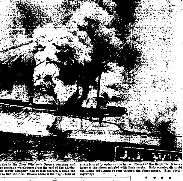
Firemen fighting fire in the Zion Wholesale Grocery company and Ralph Harris grocery company warehouses from the roof of the adjoining Gem State Paper company had to look through a thick fog of smoke and steam to find the fire. Shown above is the huge cloud of steam formed by the water on the hot ventilators of the Ralph Harris warehouse as the steam mingled with black smoke. Only occasionally could the linking red flames be seen through the dense smoke. (Staff photograph)
