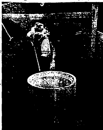
Herb Warren, one of the neighbors assisting Fran Akers in reclaiming 10 acres of land through proper drainage, here prepares to place another joint of pipe in the drainage system in place. (USDA soil conservation photo-staff gravings)
