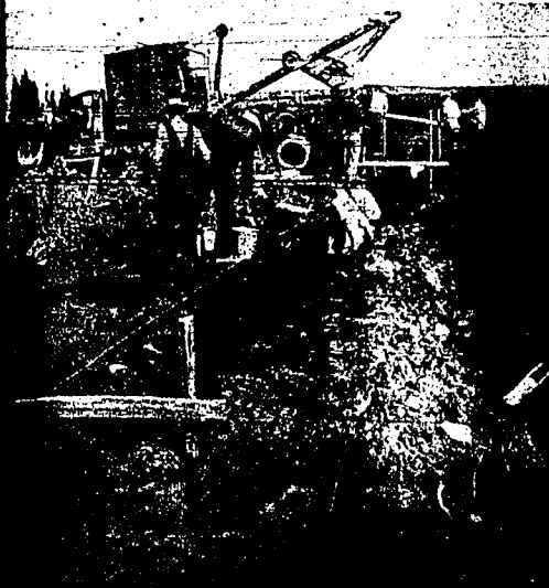
Herb Warren, one of the neighbors assisting Fran Akers in reclaiming 10 acres of land through proper drainage, here prepares to place another joint of pipe in the drainage system in place. (USDA soil conservation photo-staff gravings)
