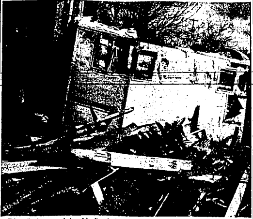
This trailer house was destroyed by fire about noon Monday while the owner, Peter Zelger, was away. Firemen are shown above as they surveyed the burned structure after carrying out the few personal articles not destroyed by the fire. (Staff photo-graving)
