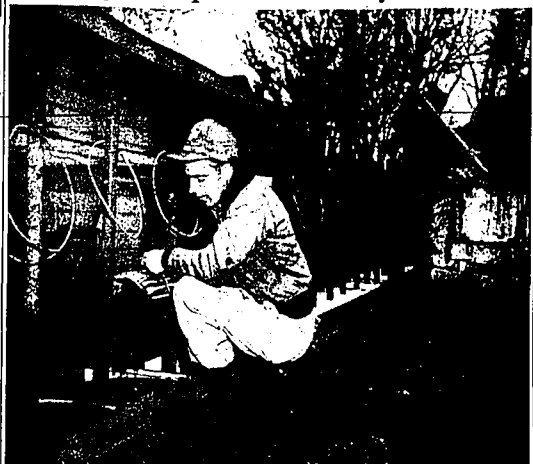
Kenneth Poe, master of the Twin Falls Grange, pours concrete into forms for rural mailbox standards which the Grange will sell to raise funds for a contribution to the physiotherapy department of Magic Valley Memorial hospital. Poe is in the background. E. T. (Pete) Crow, who's guide to point out a farmer's mailbox gives a pretty good indication of what the rest of his farm looks like. (Staff photo-entourage)
