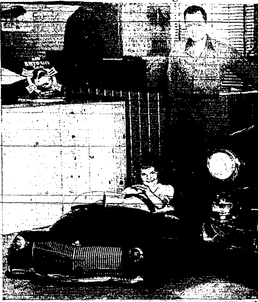
Charles McCulloch, Burley mechanic, starting with a fender from a wrecked automobile, built this sleek midget automobile for his daughter, Bonnie, 5. The vehicle, weighing 250 pounds, has a speed of 16 miles an hour. It has one speed forward and one in reverse. Most of the parts for the model car came from wrecked automobiles. McCulloch built the car in 125 hours. (Sherriff photo—staff engraving)
