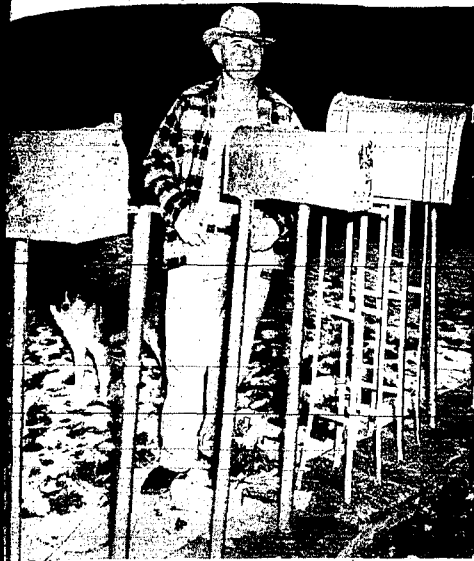
Work on modern posts being made for rural mailboxes by the Twin Falls Grange for rural mailboxes in the country. The posts, conforming to postal regulations, are four feet high and set in concrete. (Staff photo-enslaving)
