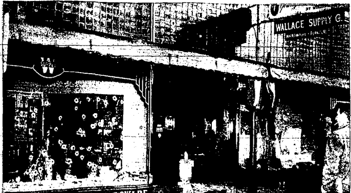
Bullets fired by police officials at a lurking gunman Wednesday morning in Wallace, splintered through show windows and tore up merchandise inside this hardware store. The store was closed for two days while workers cleaned up debris and put stocks in order. The man, identified as John Stoddard, 49, died of wounds received in the battle. Previously he had killed a Wallace miner, Gordon Hallsstone, and wounded another. Fear while burglarizing the store was advanced as the probable cause of Stoddard's action. (AP photo)
