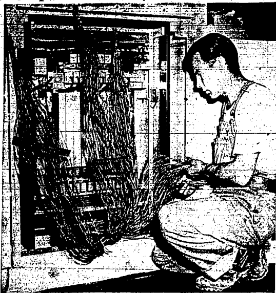
Persons placing telephone calls to Magpie Valley Memorial hospital will get the right number on each of the 78 telephones to be served by the 404 wires in this connecting cable, E. E. Ogren, switchboard installer, confidently predicts. It's no puzzle to him. About 20,000 feet of connecting wires splice the hospital switchboard to the main line. (Staff photo-gravings)
