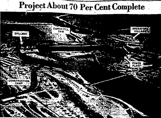
Construction on the C. J. Strike dam and power plant near Mountain Home is about 70 per cent complete. It is the Idaho Power company's sixth power plant development since 1945. The first of three generators is scheduled to be ready for operation in December. 1961. The first of three generators is scheduled to be ready for operation in December, 1961. The first of three generators is scheduled to be ready for operation in December, 1961.
