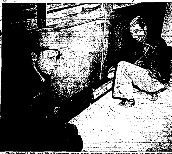
Clyde Metcalf, left, and Blair Thompson, sheet metal workers, install baseboard heating system which will be used on the top floor of the new city hall. Pipe beneath the floors will heat the lower level or basement and the ground floor. (Staff photo-ensaving)
