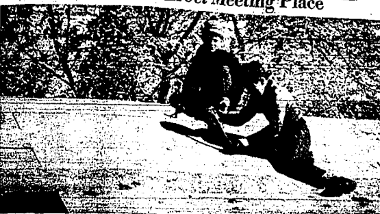
Members of troop No. 1, Buhl Boy Scouts, are erecting their own meeting place. Material for the 18-by-20-foot cabin was furnished by the Buhl Rotary club, sponsor of the troop. The cabin is located in a remote corner of the field, and is being used as a meeting place for the troop. Here a couple of the members of the troop pause in their work, while perched on the roof of the new cabin. (Staff engraving)
