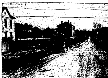
The gravel road became popular in the early 1920's. It offered a firmly packed surface, but had to be patched.
