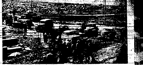
Here is a portion of parking area required for hundreds of autos.
