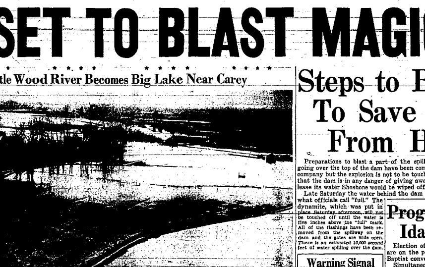
Steps to be Taken To Save Structure From High Water... Preparations to blast a part of the spillway on Magic dam to prevent the water from going over the top of the dam have been completed by officials of the Big Wood river canal company.
