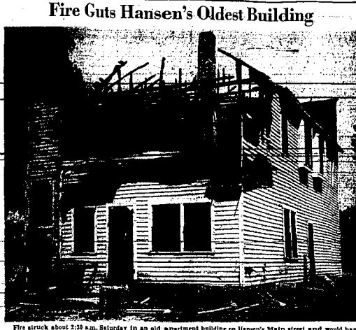
Fire struck about 2:30 a.m. Saturday in an old apartment building on Hansen's main street and would have razed the structure except for quick action by volunteers and the Kimberly rural fire department. The front of the building was damaged by fire but ruined by smoke and water. No one was living in it at the time. (Staff photo—engraving)
