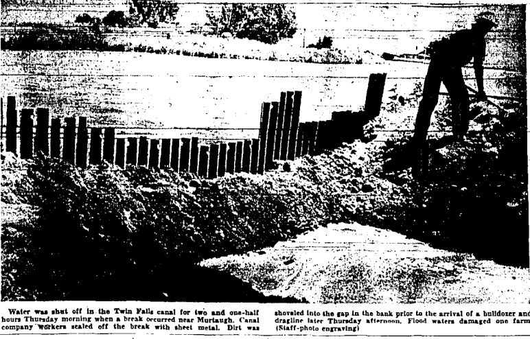
Water was shut off in the Twin Falls canal for two and one-half hours Thursday morning when a break occurred near Murtaugh. Canal company workers staked off the break with sheet metal. Dirt was shoveled into the gap in the bank prior to the arrival of a bulldozer and dragline later Thursday afternoon. Flood waters damaged one farm. (Staff-photo engraving)
