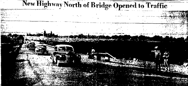
The new highway from the Perrine Memorial bridge to the Y east of Jerome was opened officially to traffic Thursday morning. Road barricades were torn down and cars moved across the new section at 9:15 a.m. Seal coating of the road will begin in approximately two weeks, according to H. B. Stenberg, district highway engineer. (Staff photographing)
