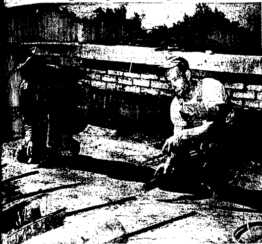
Roof repair work on the roof of the Twin Falls high school building are expected to be finished prior to school Sept. 2. Cleaning portions of the roof slated for repair are John Rogers, Jr., left, and Guy Griffith. (Staff photo-enslaving)
