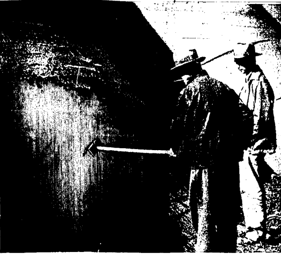
Raymond J. Briggs, consulting engineer, left, and Robert M. Nelson, both Boise, demonstrate how to apply emulsified asphalt to the surface of the Carey Valley Reservoir dam.
