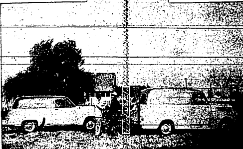
Pictured above: Our modern, portable field testing Television plant, with its 90-foot folding tower, which enables us to find the proper location and height in which TV signals are best received at your home before installing your aerial or set.
