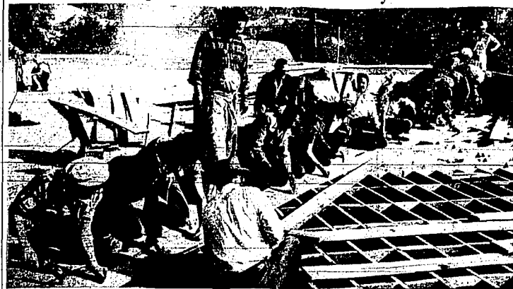
Women members of the Kimberly Methodist church took up hammer and nails to speed the construction of their new church. Here they are helping to lay the sub-floor in the building. On Tuesday the whole congregation joined in putting on the roof so the building can be enclosed before real cold weather arrives. The church was started last December and the Rev. Vernon L. Taylor, pastor, hopes to be able to dedicate the structure on Easter. (Keiker photo—staff engraving)
