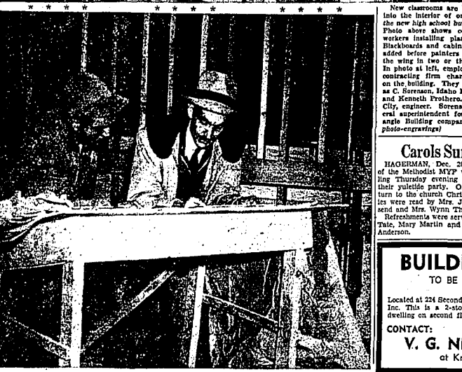
New classrooms are being built into the interior of one wing of the new high school building shown. Photo above shows construction workers installing plaster board. Blackboards and cabinets will be added before painters move into the wing in two or three weeks. In photo at left, employees of the contracting firm check progress on the building. They are Thomas G. Sorenson, Idaho Falls, right, and Kenneth Froehner, Salt Lake City, engineer. Sorenson is general superintendent for the Tri-angel Building company. (Staff photo-engravings)
