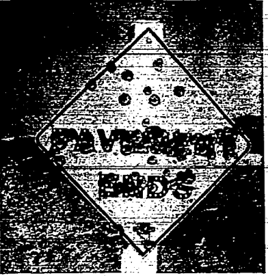
These, as left is typical of the damage to highway signs in Nevada before the department of highway started attaching targets to the signs.
