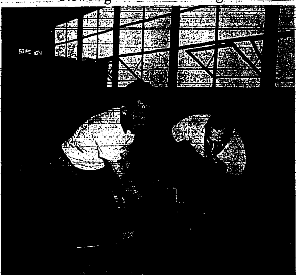
Installation of floor covering at the new Twin Falls high school building is expected to be complete in approximately 15 days. Robert Foster left and William Blakely, both Twin Falls, apply the floor covering in the chemistry room of the new building. (Staff photo-engraving)
