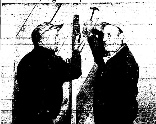
B. R. Ches, left, and Don Blackwell, help renovate the building the Dave Davis American Legion post at Carey has leased as a Legion "home." Furniture for the two rooms is being donated by Legion members and renovating includes painting, laying floor coverings and eliminating unused doorways. The work is being supervised by Keith Justison, post commander. Meetings previously were held at the high school. The first meeting in the new hall is slated for Wednesday. (Staff photo—retraying)
