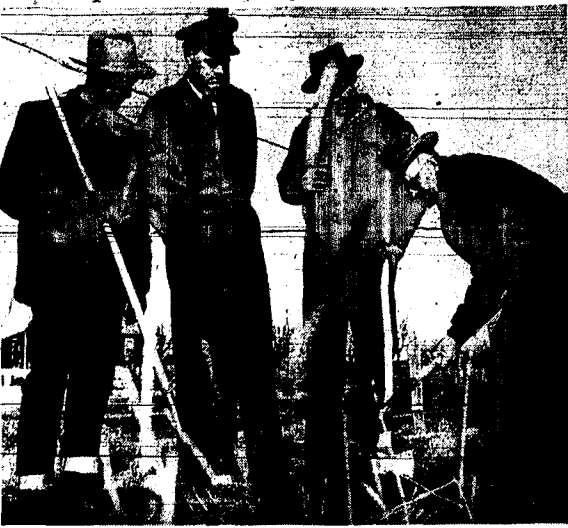
Ground-breaking ceremonies for the Hansen-Kimberly ground observer corps tower are held at a site on route 30 one mile west of Hansen. Left to right are Theodore Surrill, Kimberly; T/Sgt. Richard Dube, ground observer sector sergeant, Twin Falls; Reed C. Johnson, Hansen, chief observer, and Norville Reynolds, Hansen, post supervisor. (Staff photo-Engraving)
