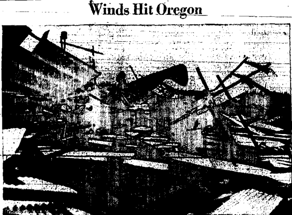
Winds up to 75 miles per hour tore these steel hangers apart and wrecked VVA planes at Troha Air park in Portland, Ore. Sixteen other planes came through undamaged when the hangers they were housed in blew apart. Damage was estimated at $50,000. (NEA telephoto)
