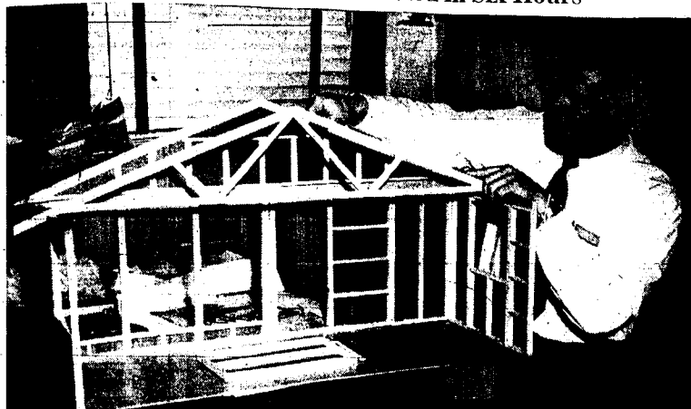
Warren Berry, manager of the Twin Falls office of Volvo Cinder Products, sets up model of firm's new panel type house which is being shown for the first time in Magic Valley. It is expected that cost of the average home will be cut by at least $500 or 50 cents per square foot of floor space. Sections of the house are prefabricated. A house can be assembled in six hours. (Staff photo-engraving)
