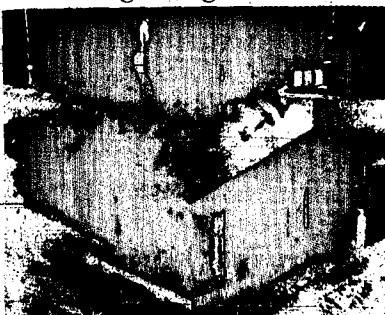
A one-story rambler home located seven-eighths of a mile from the spot where an atomic device was exploded burst into flame as the starting heat of the blast reaches Survival City, Nev. A moment later the battering force of the shock wave blew it apart. This is the second in a series of three pictures showing the home's destruction. (AEC photo via AP wirephoto)
