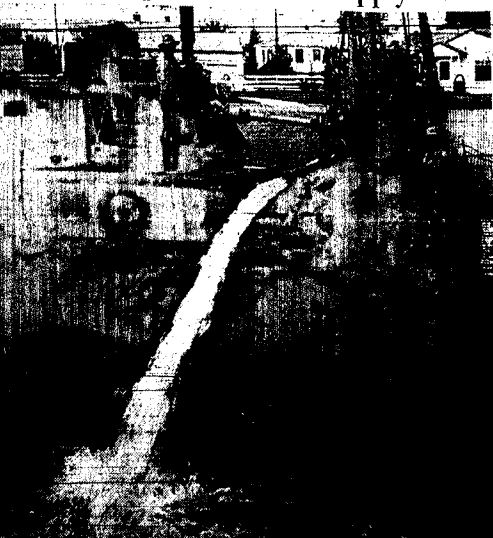
Crew from Harry Bolton Well Digging contractors struck water pumping at about 270 gallons per minute in the Willow Lane park Saturday. Here running into Ferris coulee, the water this summer will be pumped into the city system to supplement Twin Falls water supply. (Staff photo-engegraving)
