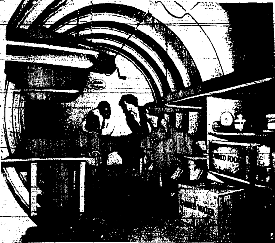
This is the interior of H-bomb steel shelter erected in Garden City, N. Y., whose developers say will take care of a family three to five days. This deluxe model is equipped with five bunks and air mattresses. At rear of tank is fan which draws pure air from outside. The handle is used in event of power failure, which also would necessitate use of battery-powered lanterns. Shelter also has radiation detector, electric battery radio, protective clothing, blankets, crowbar and shovel, first-aid equipment plus other apparatus and supplies needed to sustain family. (Staff photo-enzaving)
