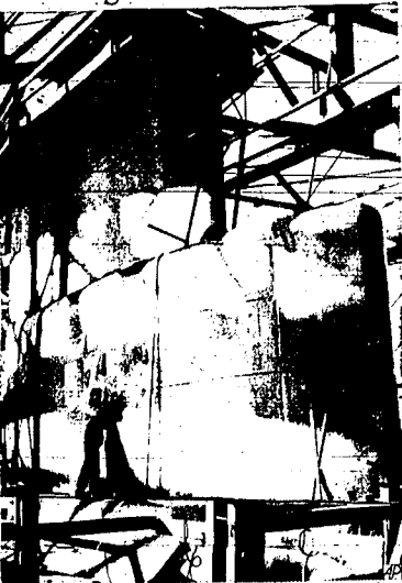
The conning tower of the Seawolf, the U. S. navy's second nuclear-powered submarine, gets her new "hat" in mid-July at Groton, Conn. The Seawolf is under construction at the Groton yard of the electric boat division of General Dynamics corporation where the nation's first atom sub, the USS Nautilus, was launched nearly 18 months ago. The two ribs are much alike externally, but there is a difference in the atomic reactor propulsion plants. (AP wirephoto)
