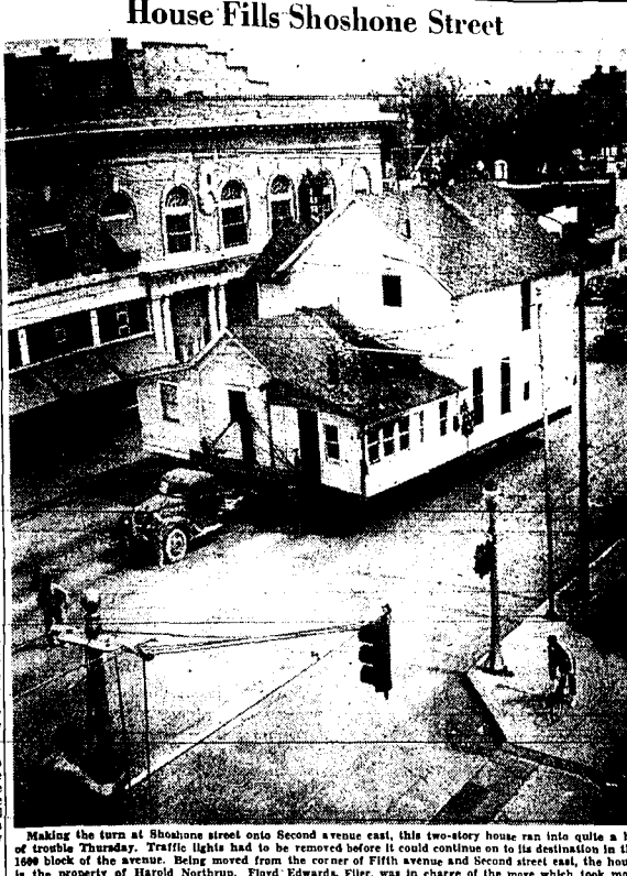
Making the turn at Shoshone street onto Second avenue east, this two-story house ran into quite a bit of trouble Thursday. Traffic lights had to be removed before it could continue on to its destination in the 1500 block of the avenue. Being moved from the corner of Fifth avenue and Second street east, the house is the property of Harold Northrup. Floyd Edwards, filer, was in charge of the move which took more than a day to complete. (Staff photo-entourage)
