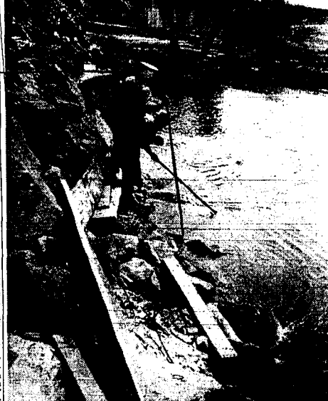
Idaho highway maintenance men keep the three nine-foot pipes under the fill at highway 36 near Mario Valley Memorial hospital open and free of logs and debris as flood waters rushed down Rock creek canyon Friday night and Saturday. (Staff photo-engraving)
