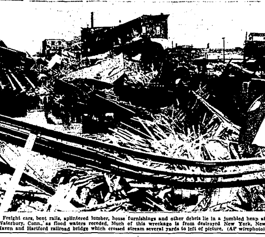
Freight cars, bent rails, splintered lumber, house furnishings and other debris lie in a jumbled heap at Waterbury, Conn., as flood waters receded. Much of this wreckage is from destroyed New York, New Haven and Hartford railroad bridge which crossed stream several yards to left of picture. (AP wirephoto)
