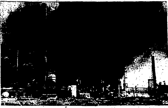
Little more than a tangle of pipes and tanks remains where formerly stood the 26-story hydroformer cracking tower in area just to right of tall chimney at the Standard Oil company, of Indiana's Whiting, Ind., big refinery. The hydroformer disintegrated in an explosion which set fire to vast stores of oil and gasoline. The multi-million dollar base was under control today. (AP Wirephoto)
