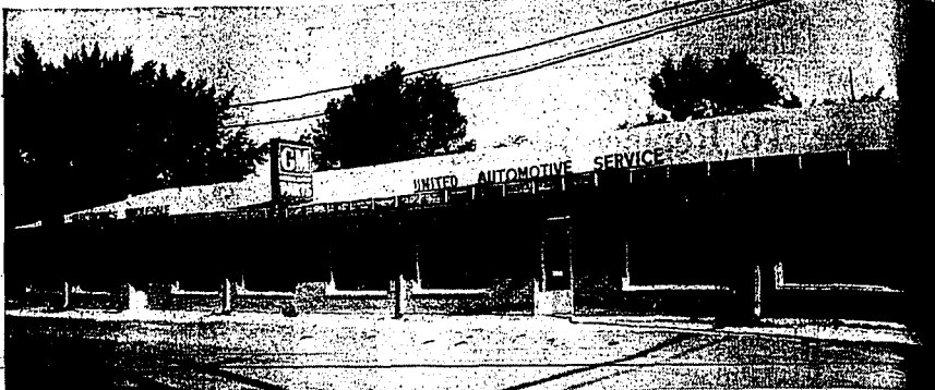
New Home of United Automotive, at 228 2nd Street East, Twin Falls, just completed by Mr. and Mrs. Reed Goold, to house their enlarged Automotive Parts business and their complete line of Electronic Parts and equipment. This is Magic Valley's first and only Wholesale warehouse of original parts for all makes and models General Motors cars and trucks. This firm still occupies their former site adjoining, as well as this large new building which will accommodate their wholesale Electronic and their automotive parts consisting of over 200 wholesale lines.
