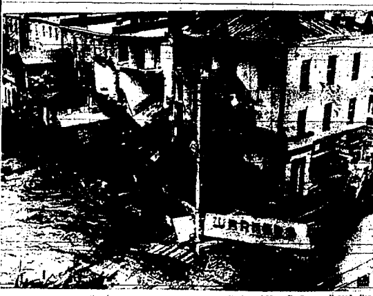
Business houses built over this downtown section of the Newhall river at Merrill, Conn., collapsed after foundations were weakened by the second flood in a two-month period. Sign in foreground is from one of the stores that was swept into the flood-swollen river leaving neighboring structures badly damaged. (AP wirephoto)
