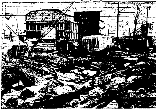
Flood-torn debris covers the New York, New Haven and Hartford freight yards in Norwalk, Conn. After the ravaging waters receded, Connecticut was the hardest hit of seven northeastern states from hurricanes and floods that took 50 lives, threw 25,000 y-crooks over the edge and damaged was estimated at $500-million. (NEA telephoto)
