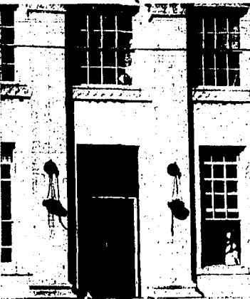
An unidentified passerby looks into postoffice building in Gettysburg, Pa., where women in window at right are renovating an office to be used by President Eisenhower during his stay on his farm near here. (NEA)
