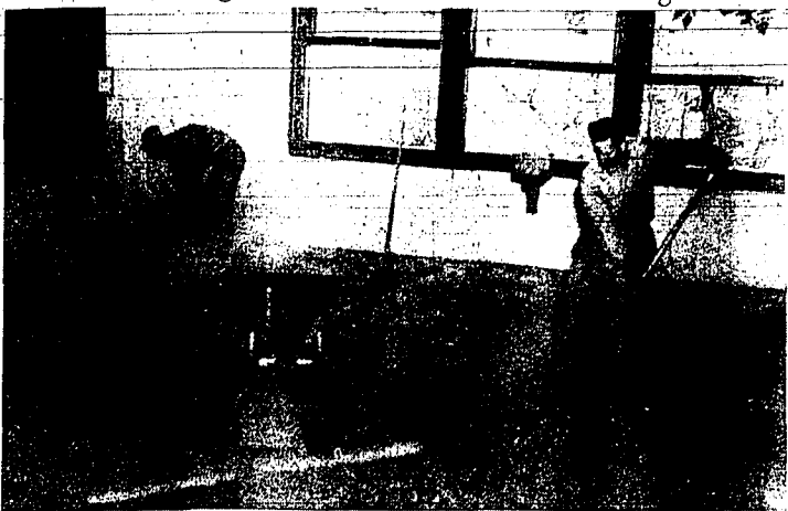
Barely visible through the dust in the chemistry laboratory, Roy Kinney, left, and John Rose, remove the first shovelful of an expected 52 1/2 tons of concrete flooring to be taken from two condemned rooms in the junior high school. With the concrete on the physics room floor, Owen Kinney, building inspector, estimates that a total of 52 1/2 tons will be removed. Kinney said the laboratory flooring had settled about three inches in the center. Work was expected to be completed Tuesday. (Staff photo-enraving)
