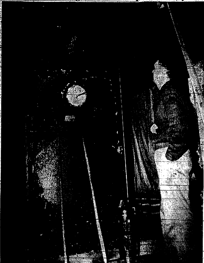
Verns Elstinger, hatchery man for Swift and Company hatchery and feed store, 347 Main avenue east, inspects damage to one of the electrical incubators following Sunday fire. The fire, believed started by defective electrical wiring swept the interior of the plant Sunday afternoon. Twin Falls firemen brought the blaze under control within 17 minutes, keeping the fire within the building. (Staff photo-engraving)
