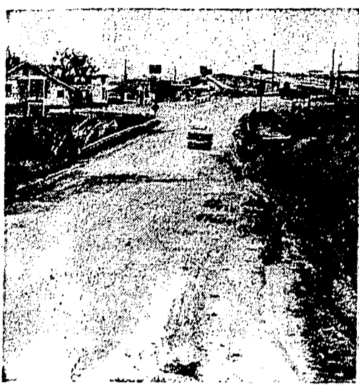
and high speeds cause the pavement to break. Highway department officials anticipate one of the worst breakup seasons in recent years. Maintenance crews are working to keep the surface in the safest travel condition. Note warning signs at edge of road in photo at right.
