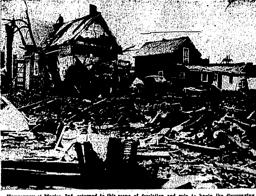
Homeowners at Marion, Ind., returned to this scene of desolation and ruin to begin the discouraging task of clearing away debris, patching roofs and rebuilding houses. Several persons in these two houses were injured when the tornado struck. One person in Marion was killed. (NEA telephoto)
