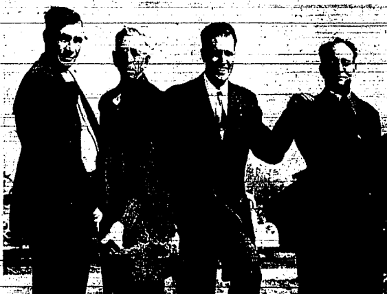
Members of the Southern Baptist church began their church building program with a brief groundbreaking ceremony Sunday afternoon. The new building will be erected on the southeast corner of Filer avenue and Washington street, north and will be of frame construction with brick veneer finish. Above Earl Massey, church treasurer, left, and
