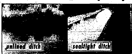
Actual photo of lined ditch. High water-level due to seepage and rodents. Weed growth and moss slows water movement. Unretouched photo of Sealtight-Morse ditch in Yakima Valley. Water-flow is rapid. Note absence of weed growth.
